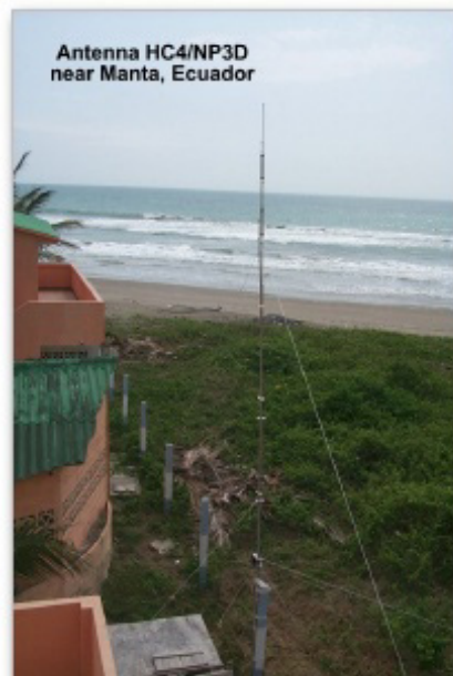
Antenna HC4/NP3D near Manta, Ecuador
